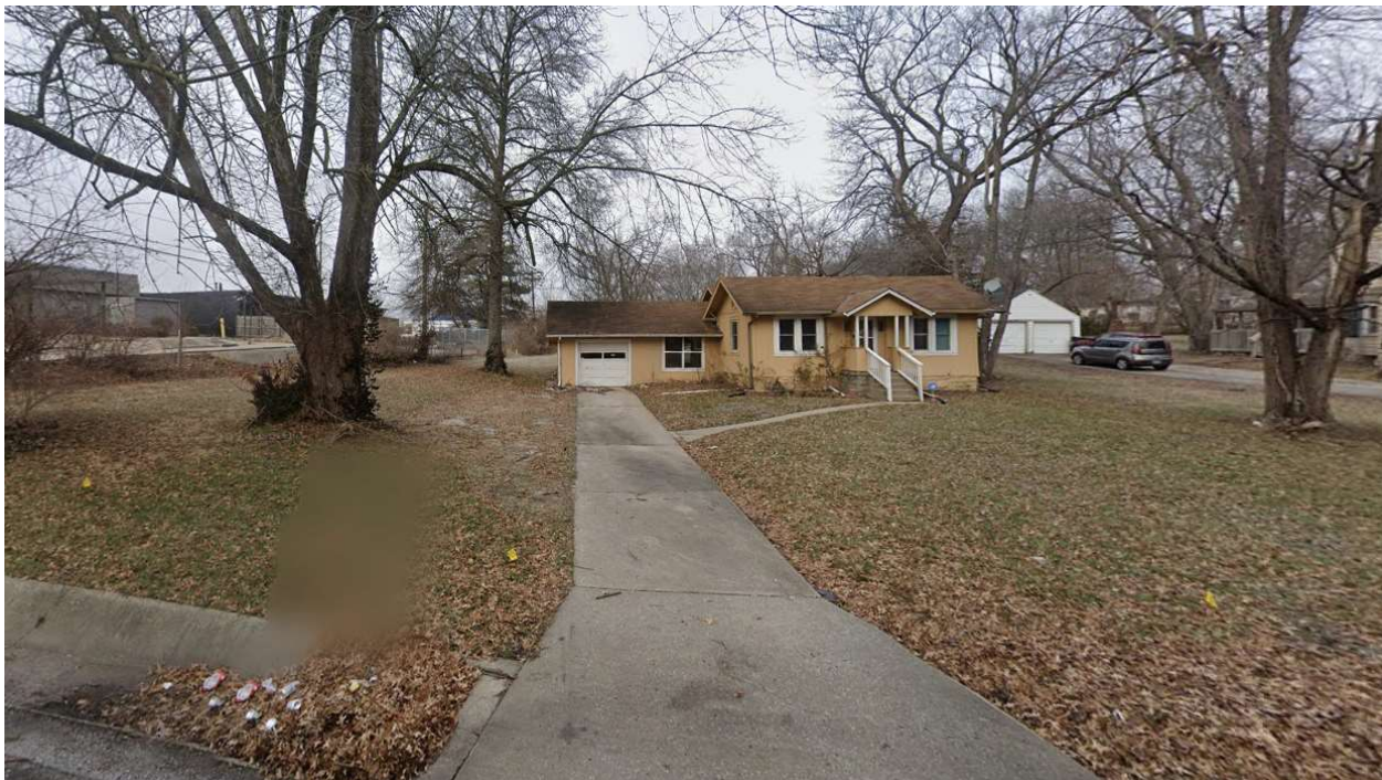
Facing 6920 Laurel Ave. (vacant residence)
